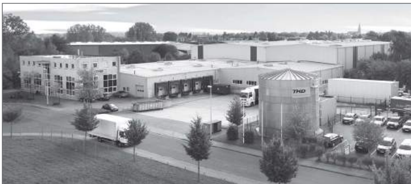
TKD centro logistico Nettetal / TKD Logistics center Nettetal
